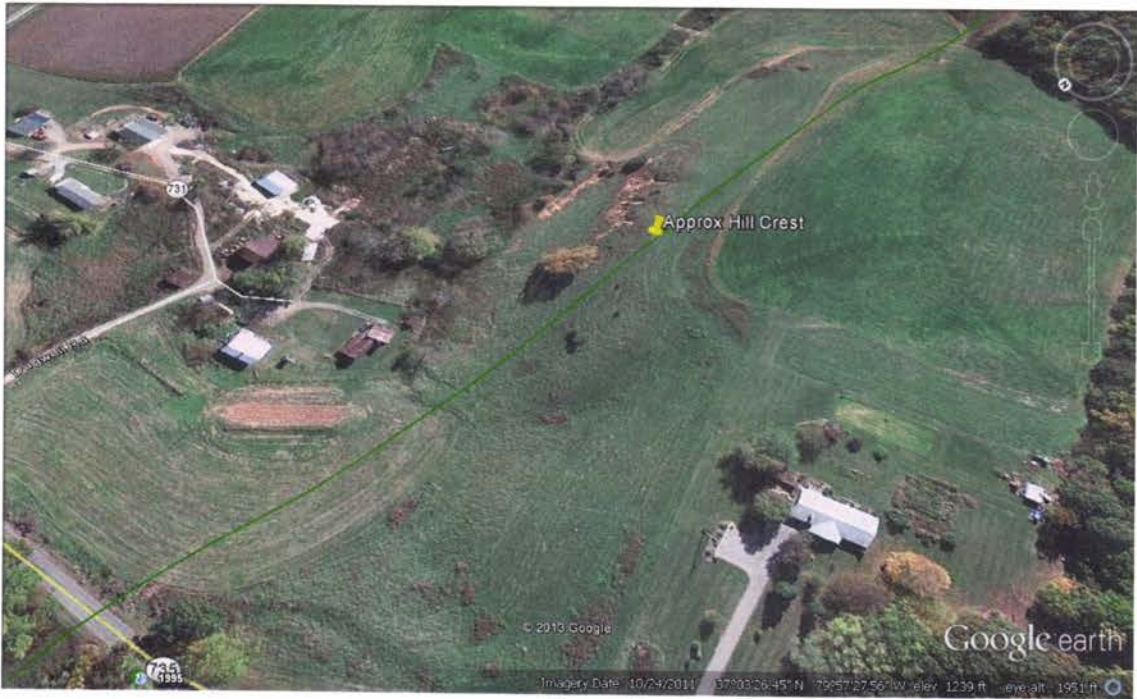
Figure No. 5 8RK pipeline crossing mowed pasture at Retreat Road
